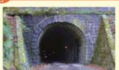
Old Amagi tunnel
